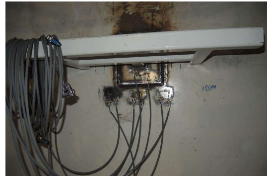
Fig. 5 – Loading console welded to the steel structure front view
