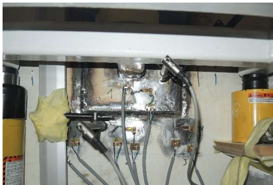
Fig. 3 – Strain gauges with electrical resistance
